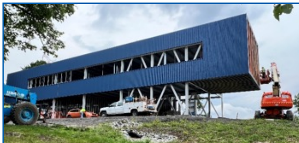
Construction of Ideal Saldi Hall, Johnson College
